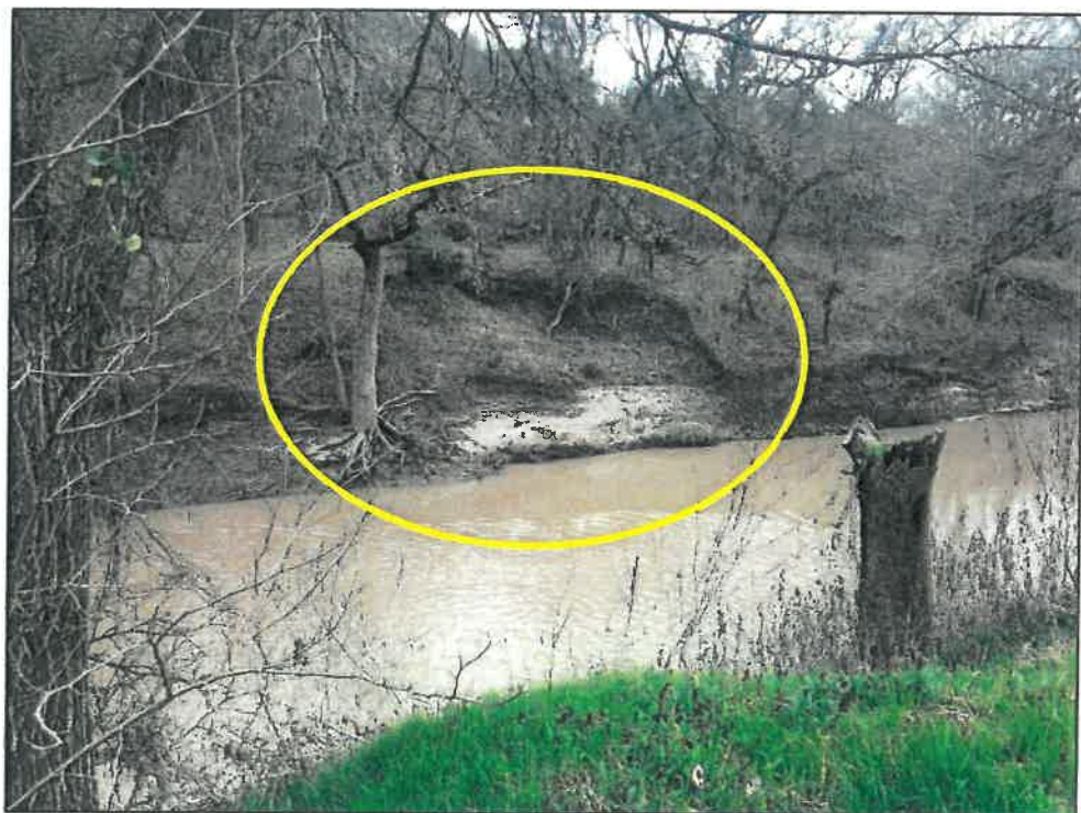
Figure 15: Leon River bank slope failure opposite Faunt Le Roy Park
